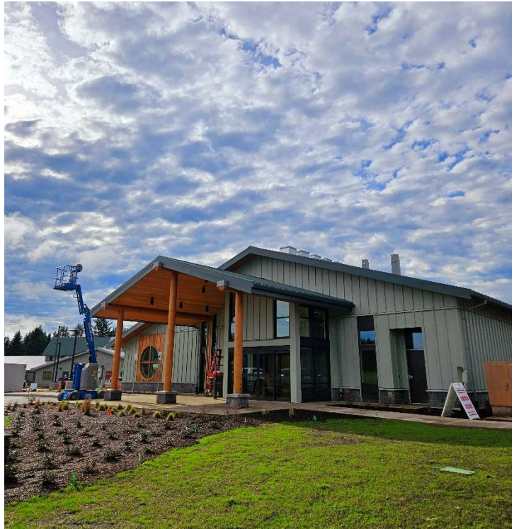
Healthcare and Vaccination Clinic under Construction, January 2024
