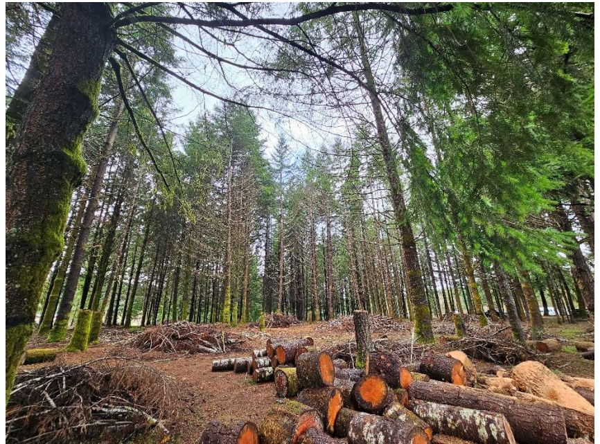
Nature Playground area being prepared for construction to occur in Spring/Summer 2024.
