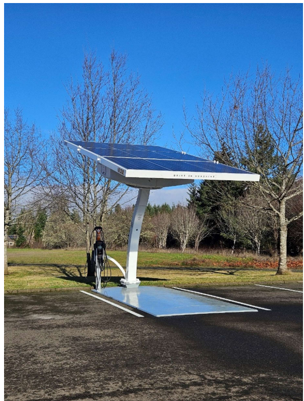
Solar Electric Vehicle Charging Station near Governance Center
