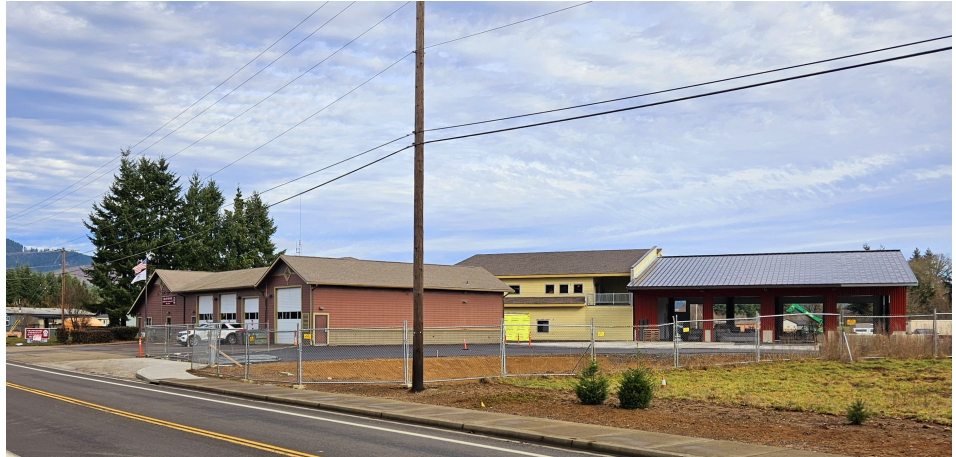
The Fire Station Expansion Project is underway, January 2024
