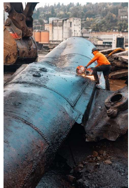
Underground Storage Tank removal at tumwata village site.
