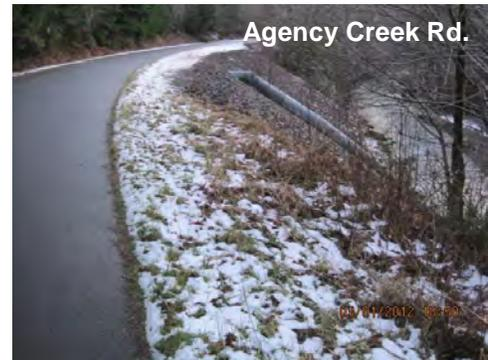
In addition, the lack of guardrail on Agency Creek Road and the steep slope high above the creek create unsafe conditions. Installation of guardrail at problem locations can reduce the risk of vehicles leaving the roadway as well as the potential for environmental impacts from chemical spills into the creek.
