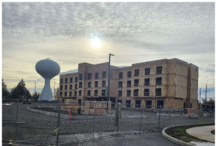
Chemawa Station – Hotel Under Construction
