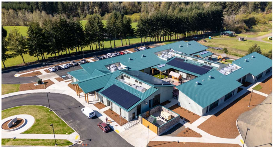
(Top) Ribbon Cutting Ceremony (Middle) Aerial Image of Completed Building (Bottom) Tribal Art & Ribbon Cutting Announcement
